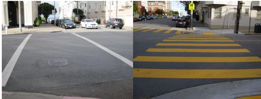
Figure 2. Two common kinds of crosswalk marking patterns. Left: two transverse lines (“two-stripe”). Right: continental (“zebra”).
