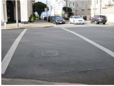
Fig. 1. The “two-stripe” (two transverse lines) crosswalk marking pattern.
